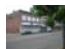
Figure 4: Neighborhood view of opposite side of Martin Luther King, Jr. Way, taken from the back of the ICC
